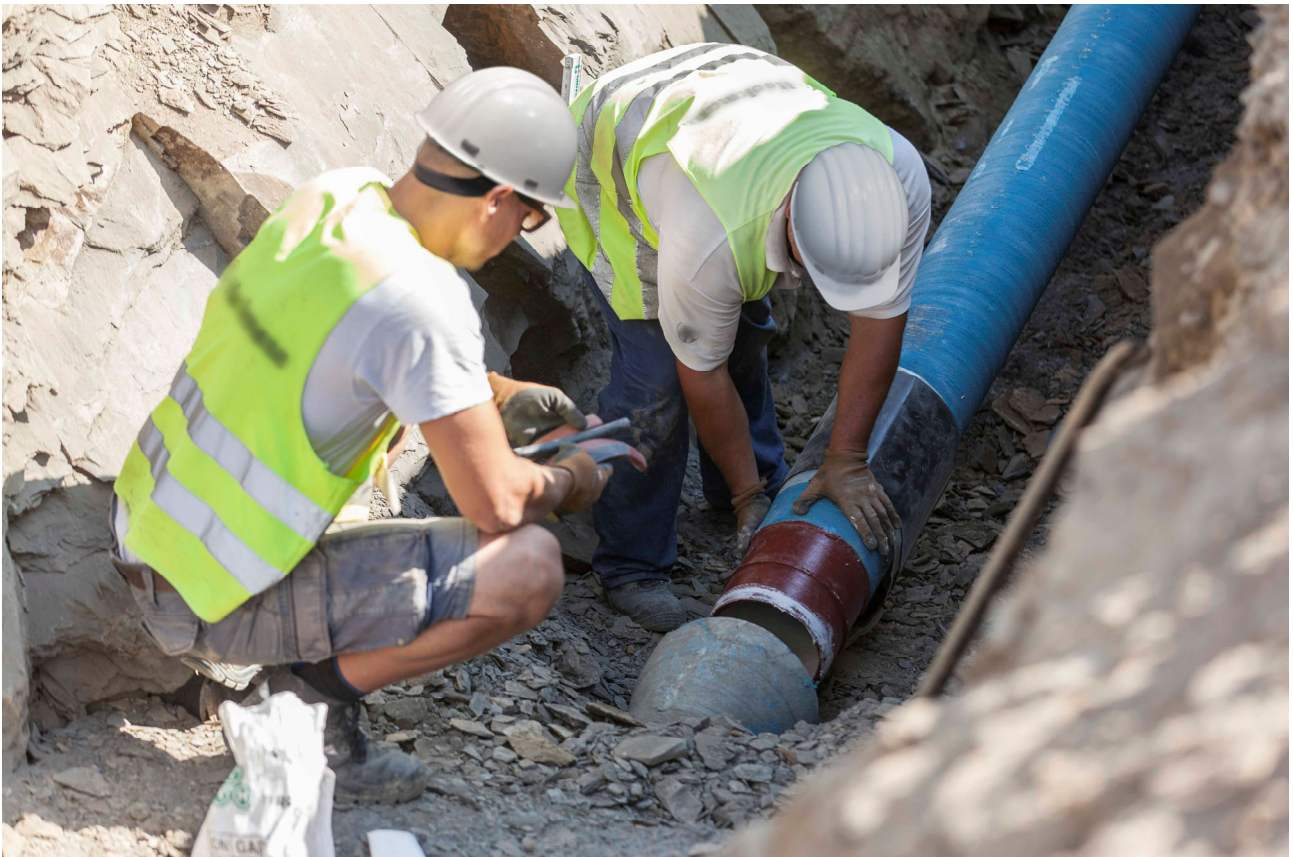
Pipeline installation/assembly in the open trench
