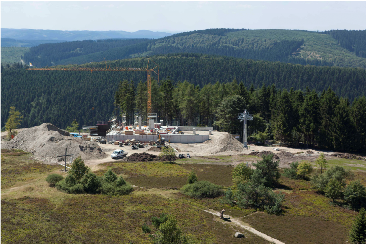
Newly constructed mountain lift station
