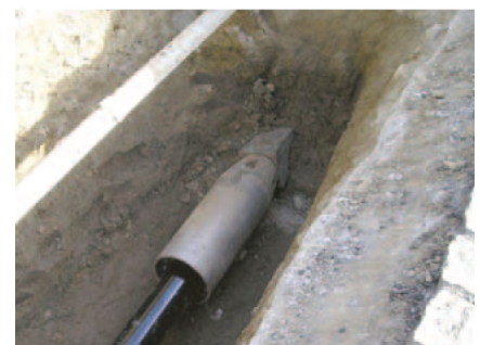
Bursting head and expanded drilling channel
