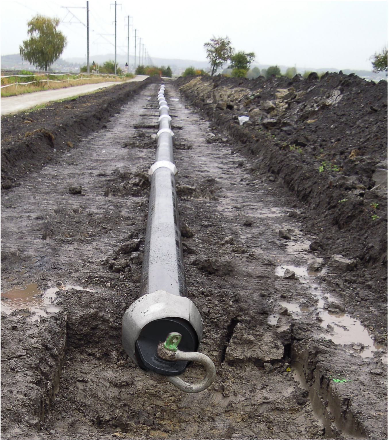
Preassembled pipeline
