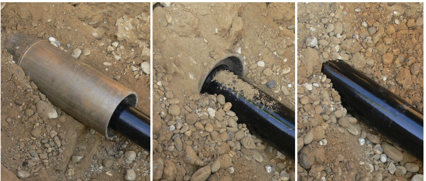
Pipe laying with ECOPUR BLS fully protected pipes
