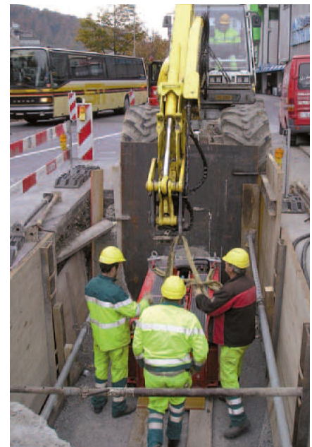
Installing the winch
